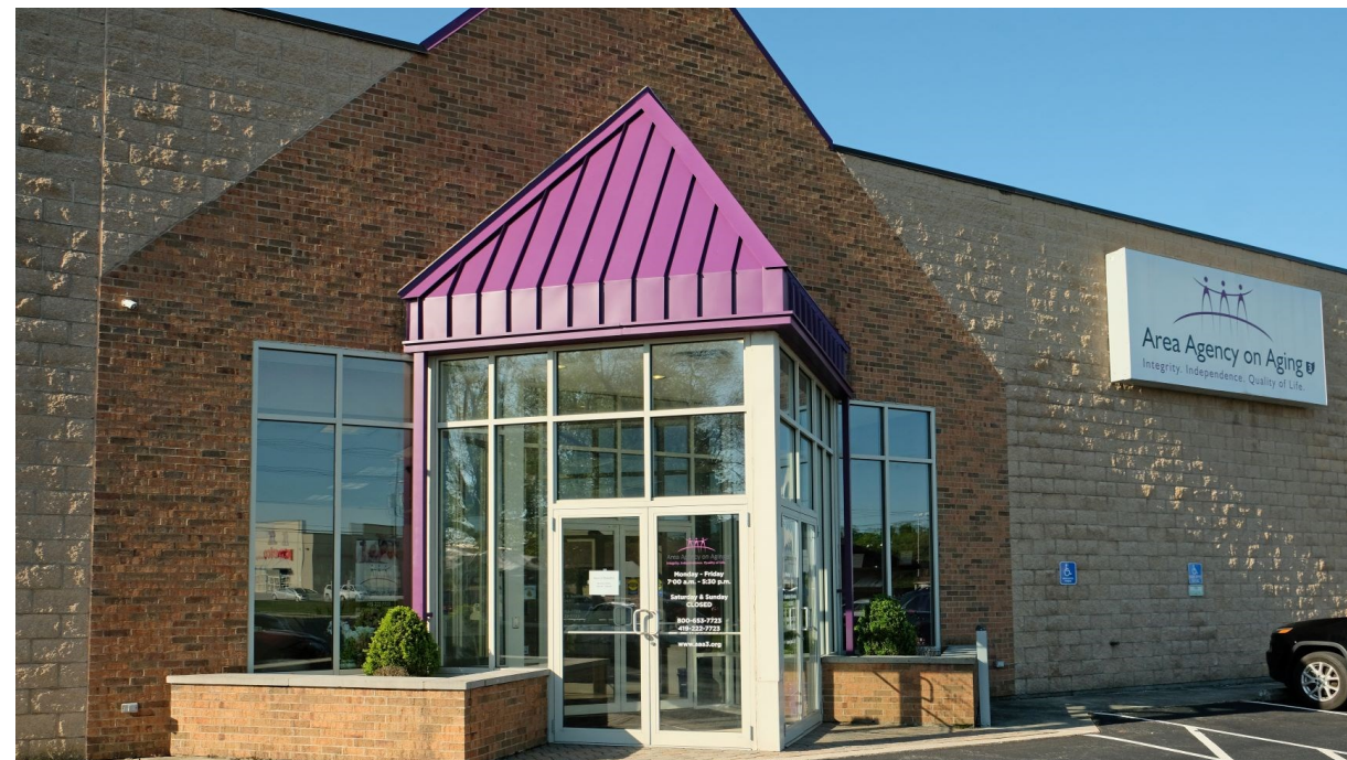
AAA3 is located at 2423 Allentown Road in Lima
